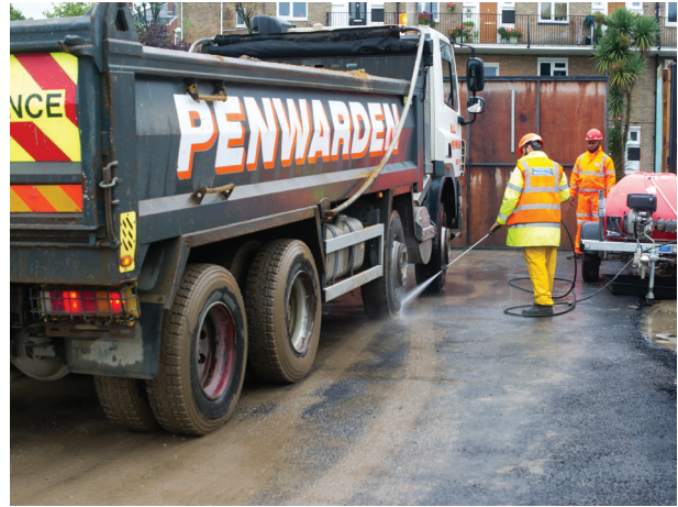
Vehicle wheels being inspected and washed before leaving site
